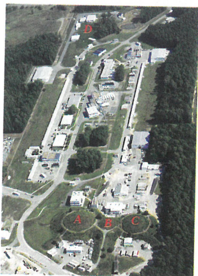
Figure 3. The CEBAF Accelerator includes two antiparallel 1-GeV linacs connected by two magnetic arcs. A beam is delivered to experimental Halls A, B, and C at 11 GeV, and D at 12 GeV. The total distance around the accelerator racetrack is 7/8 of a mile.
